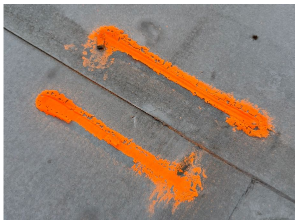
Obr. 11 Defekt B7 detail
